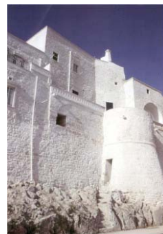
Typical white walls
